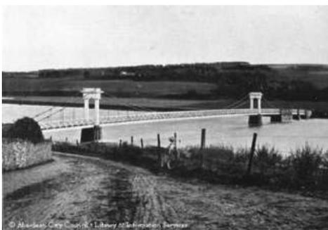
*Over the years the bridge has been damaged by floodwaters and from 1955 onwards the river shifted its course and the southern approach span was swept away. In 1984 the decking was removed as a safety precaution and the bridge is now derelict. The Community Council have*
